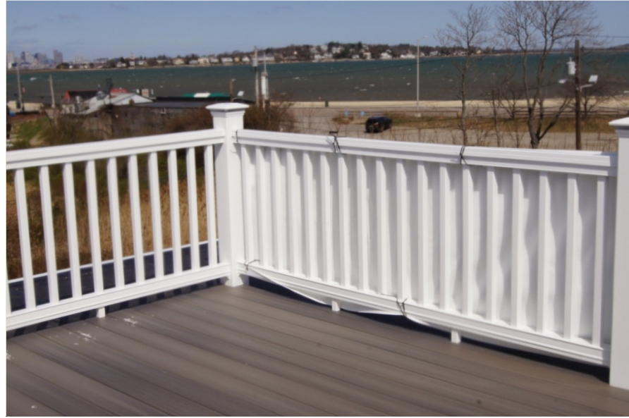
Roof Deck VIEW
